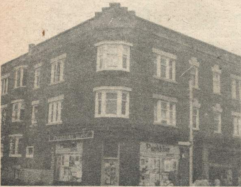
The Wineva-Queen building in happier times. Pushkin's Depot, a hip-capitalist "non-sectarian" left bookstore, continued to operate even after the building was totalled.
