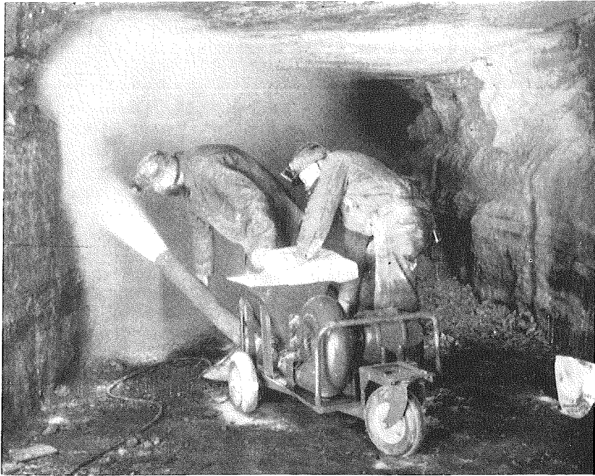
Rockdust sprayed on mine section helps prevent spread of coal dust explosion.
