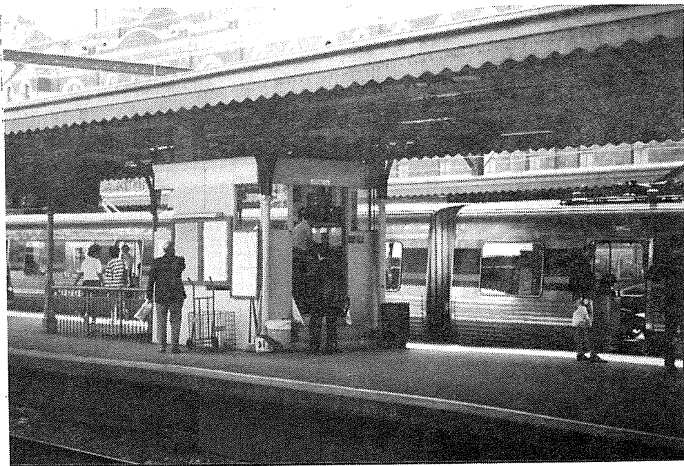
ANTIQUATED PLATFORM CABIN, FLINDERS STREET STATION.
