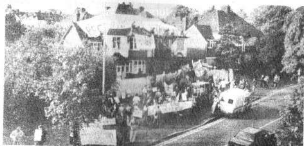
Protestors take over houses in Wanstead, East London as they resist the construction of the M11 link road which involves the demolition of 400 homes
