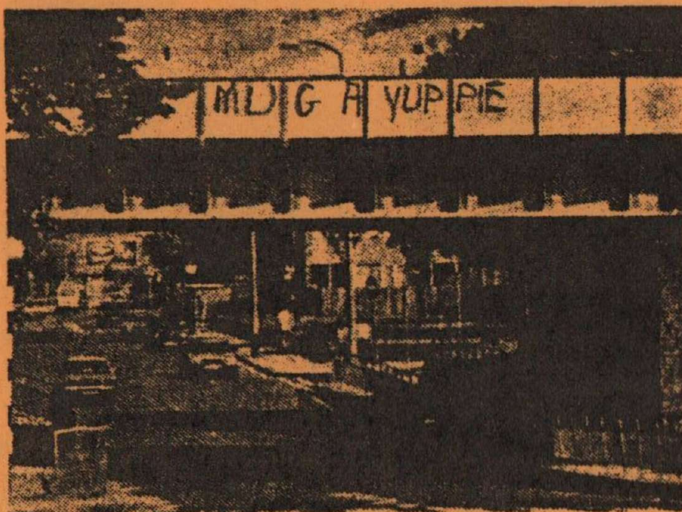
Grove Road railway bridge, Bow.
